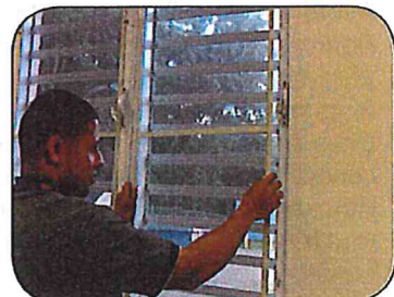
Install or repair window & door screens.
